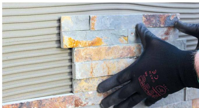
SlipBond can be applied to a thickness of 3mm-20mm and it's frost resistant.
